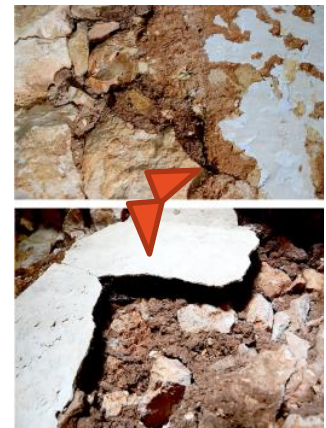
Fig. 12. Natural elements showing the thick layer of plaster; “ Hhouwara ”
