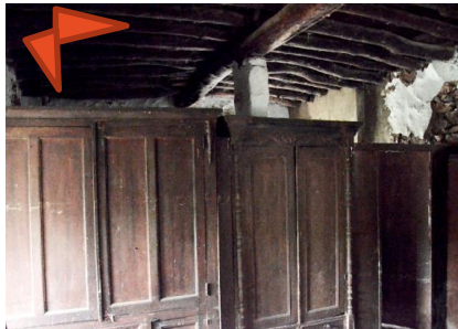
Fig. 17. ceiling made of wooden loges; “Ousallet” with a huge old “Youk” underneath
