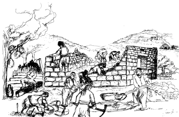
Fig. 21. My illustration showing the act of "A-aounet" in building an old vernacular house in ancient times.
