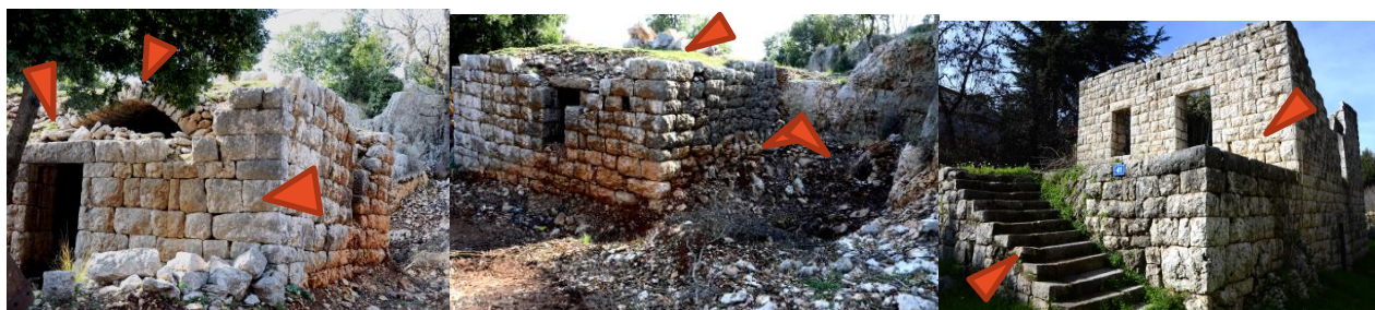
Fig. 6. My pictures of some remains of vernacular houses in Achkout showing shattered ruins or “ Khirbi ”, where there still exist; “ A-atbet ”, “ A-aed ”, “ Midmek / madamik ”, “ Satehh ”, “ Manbesh ”, “ Daraj ” and “ Staihha ”.
