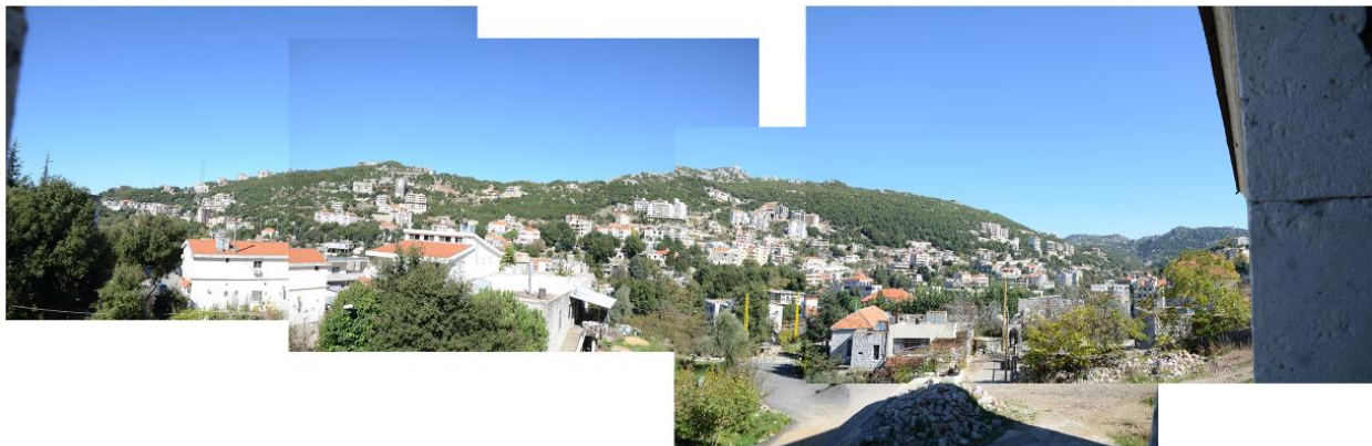
Fig. 5. Personal pictures showing the invasion of concrete, Achkout, 2018.
